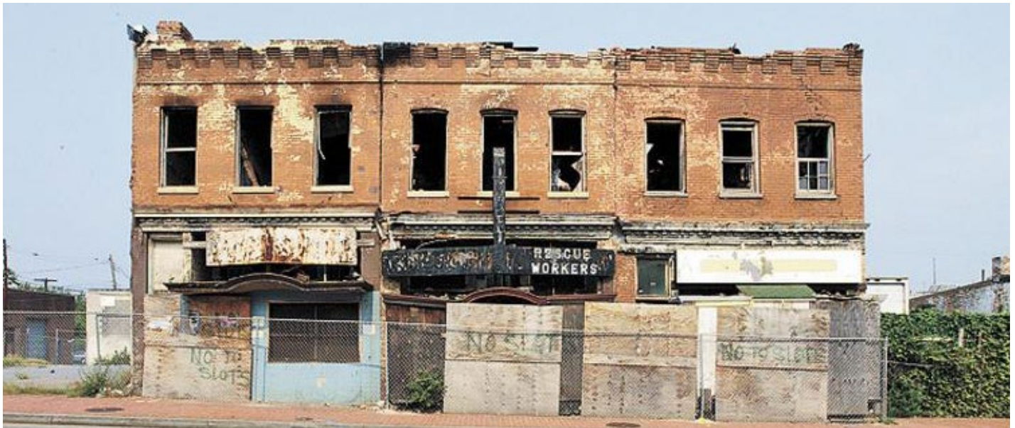
These historic buildings at 1909-1913 Martin Luther King Jr. Avenue in Washington, D.C., collapsed due to neglect in 2015 (bizjournals.com).
