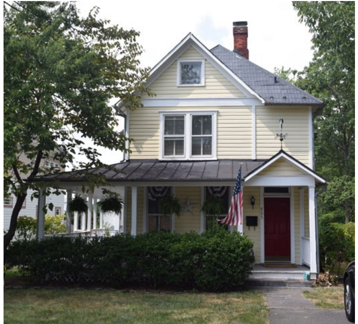
Wood clapboard or weatherboard siding, seen here at 805 Monroe Street (above) and 765 Monroe Street (below), is easily replicated and should be replaced in kind.
