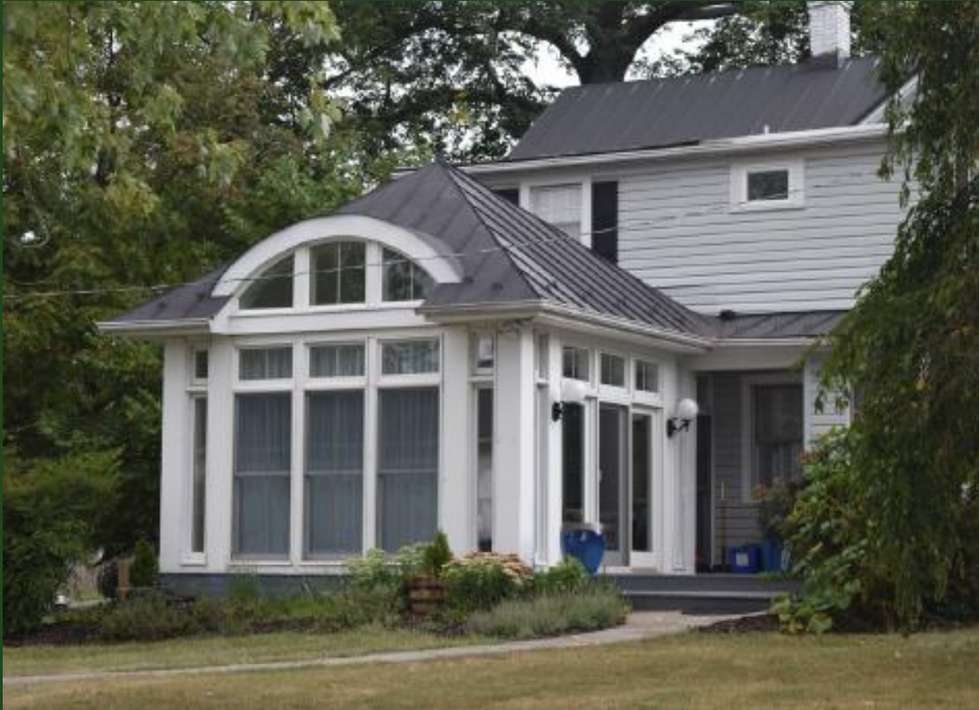
This addition to the rear of 651 Spring Street is compatible because it isn't visible from the front of the house.
