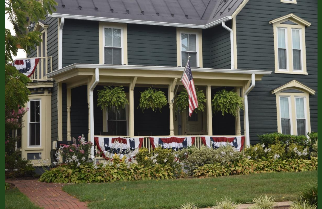
Covered porches like the one at 763 Grace Street provide shade and promote cooling.
