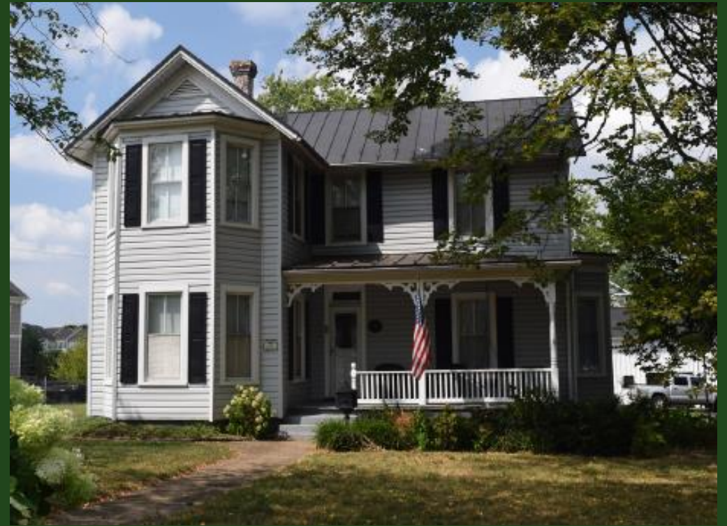
This home at 651 Spring Street retains character-defining features like the decorative porch brackets and railing, seamed metal roof, two-story projecting bay, and overall form from the front.
