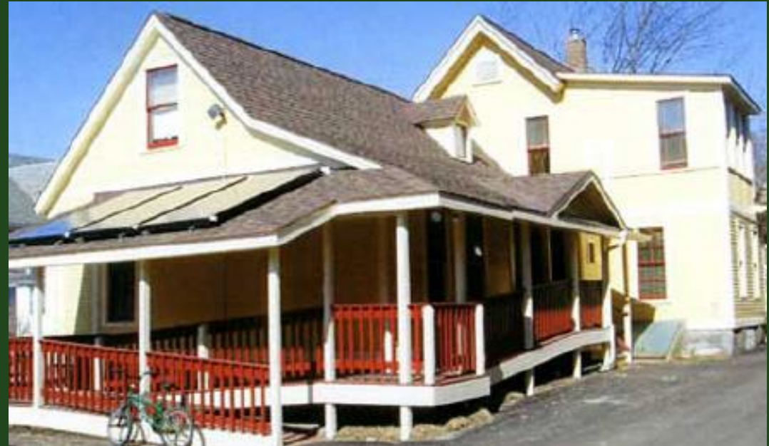
Solar panels on a historic building should always be located on a rear elevation and out of public view to avoid detracting from the building's integrity.
