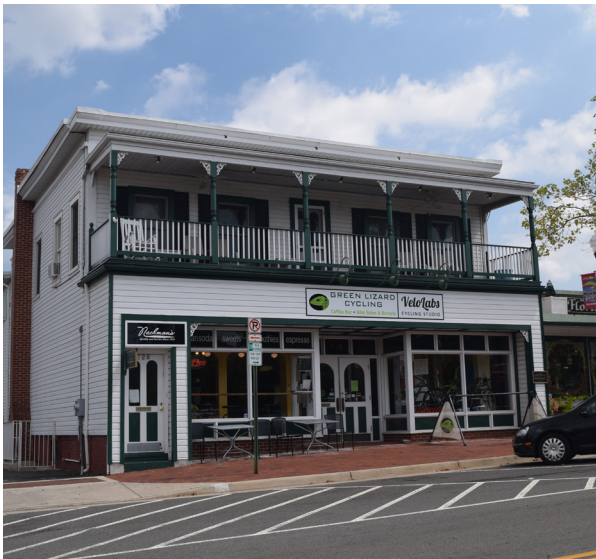
Historic buildings attract small businesses, like Green Lizard Cycling and Coffee in Herndon.
