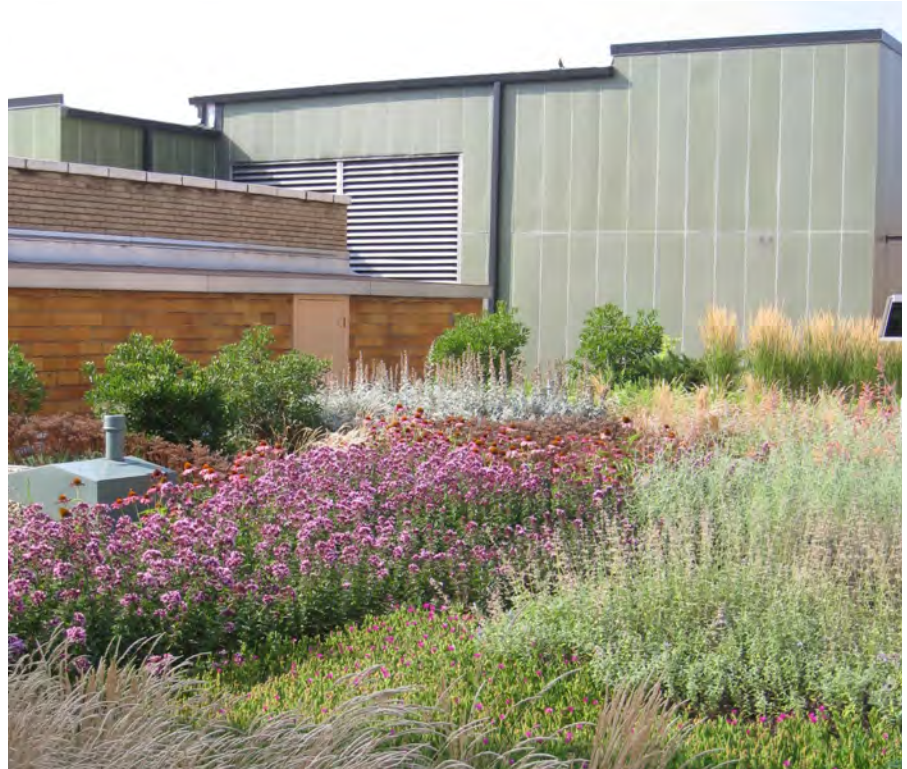
Native perennial planting on the Allegheny County Office building's green roof provide visitors with an unexpected garden.
