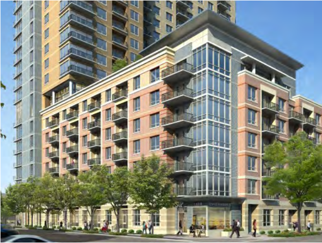
Podium Building with a Tower rising beyond
