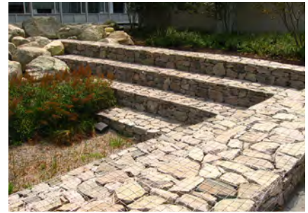
Above ground retention
