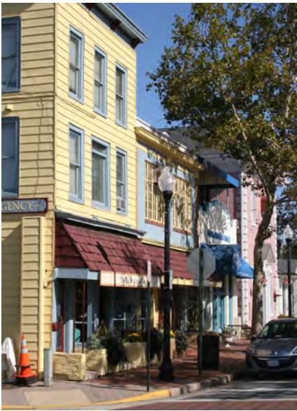
Existing historic buildings in downtown Herndon
