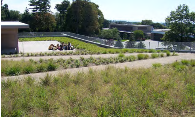
Above ground retention on a roof garden
