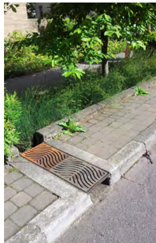
Public streets using stormwater planters to capture rainwater
