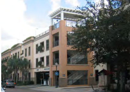
Parking structures help developers build at higher densities and in phases. Throughout the HTOC, parking structures should be designed to resemble buildings.
