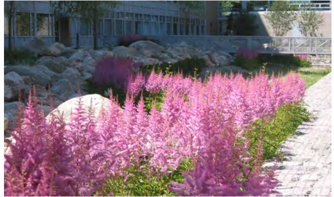
Stormwater wetlands in bloom. A variety of textures and colors provide visual interest for the pedestrian realm while allowing rainwater to slowly infiltrate.
