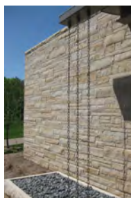
(Far left) Sub-surface stormwater retention occurs at this recessed lawn (Left) Rain chains collect water for use as harvested building grey water
