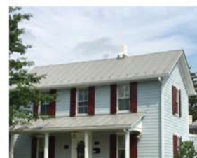
Standing seam metal roof
