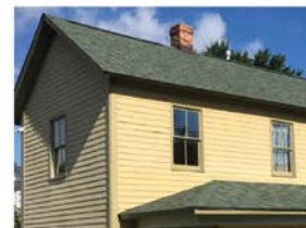
Asphalt shingle roof
