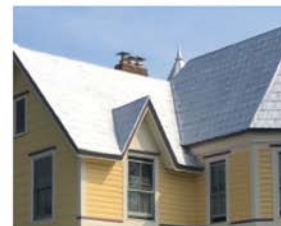
Stamped metal roof
