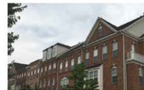
Dormers on noncontributing building
