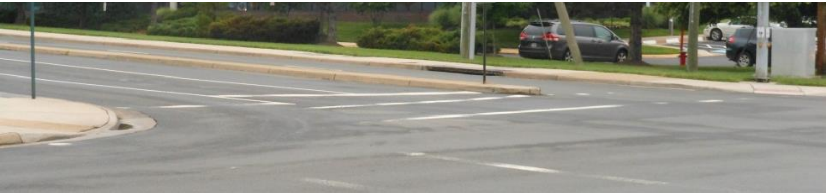
Photo of low visibility crosswalks – Located at Herndon Parkway and Spring Street
