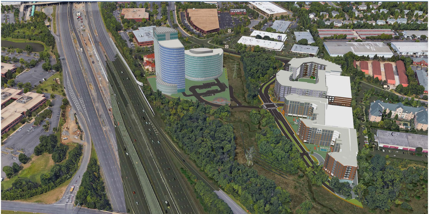
1 VIEW FROM TOLL ROAD
