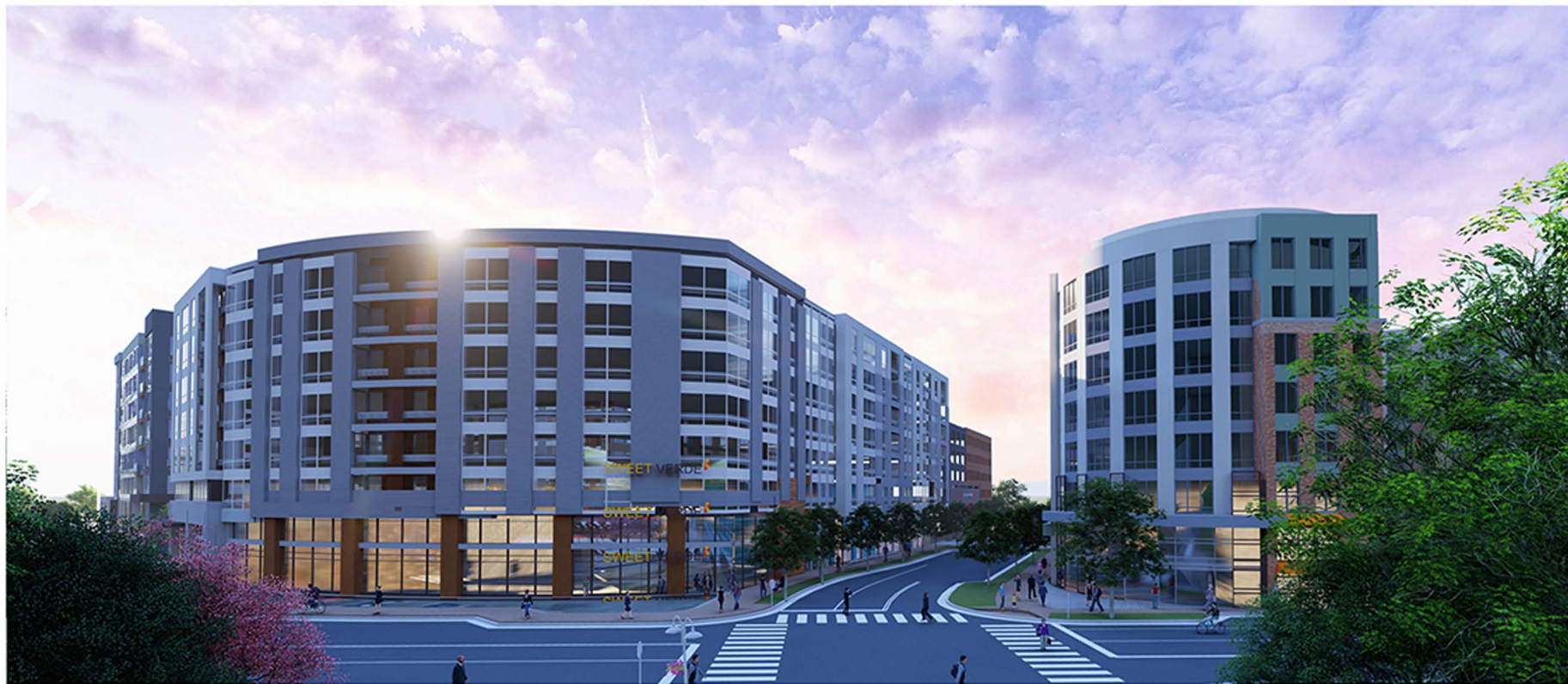
6 BUILDINGS 3 & 4 VIEW FROM FAIRBROOK DRIVE
