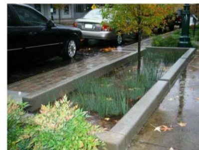
BIORETENTION PLANTERS TREAT STORMWATER FROM THE ROOF AND ARE PLANTED HERE WITH LARGER PLANT MATERIALS INCLUDING SHADE TREES, WHICH IN ADDITION TO BEING AN INTEGRAL PART OF BIORETENTION, ALSO SERVE AS STREET TREES, SHADING THE SIDEWALK AND REDUCING THE SCALE OF THE ARCHITECTURE
