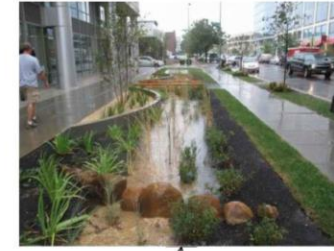
BIORETENTION PLANTERS CREATE LANDSCAPE OPPORTUNITIES ADJACENT TO PEDESTRIAN AREA AND SERVE TO TREAT STORM WATER FROM THE BUILDINGS
